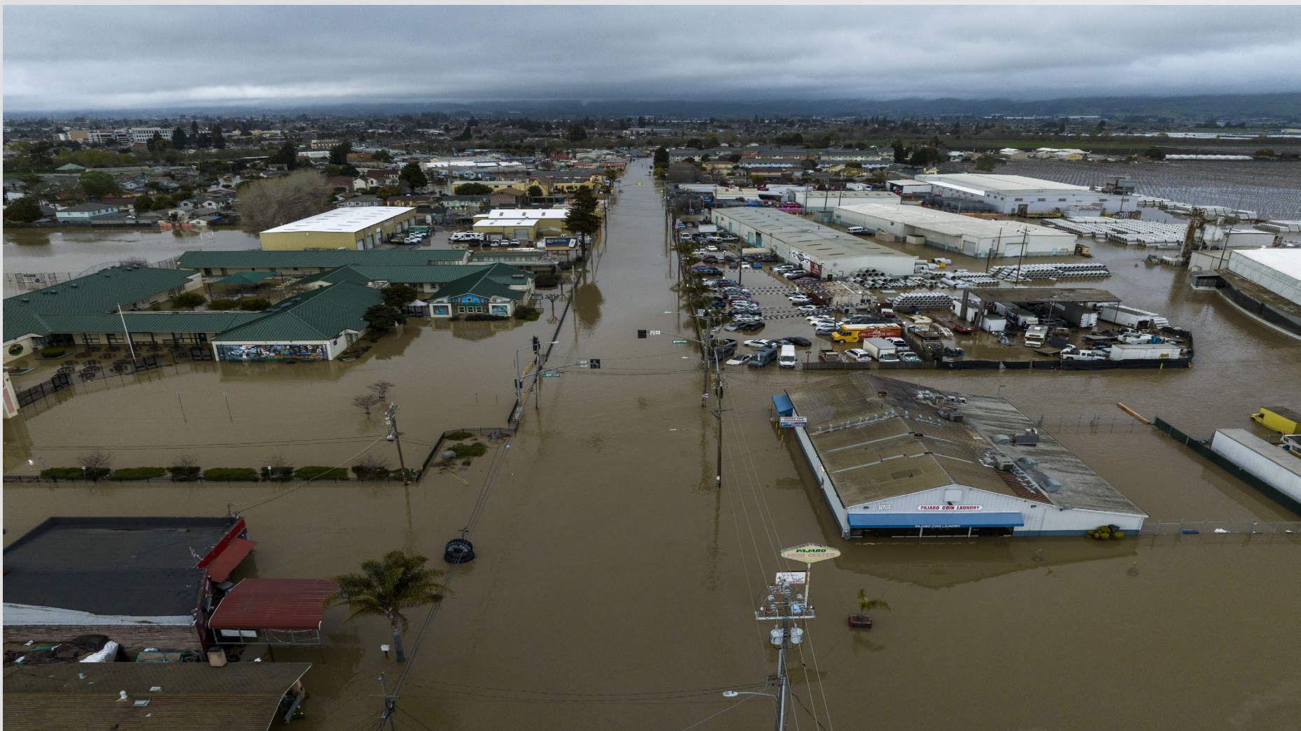
March 12, 2023, Pajaro levee breach causing extensive flooding in the Town of Pajaro of Monterey County.
