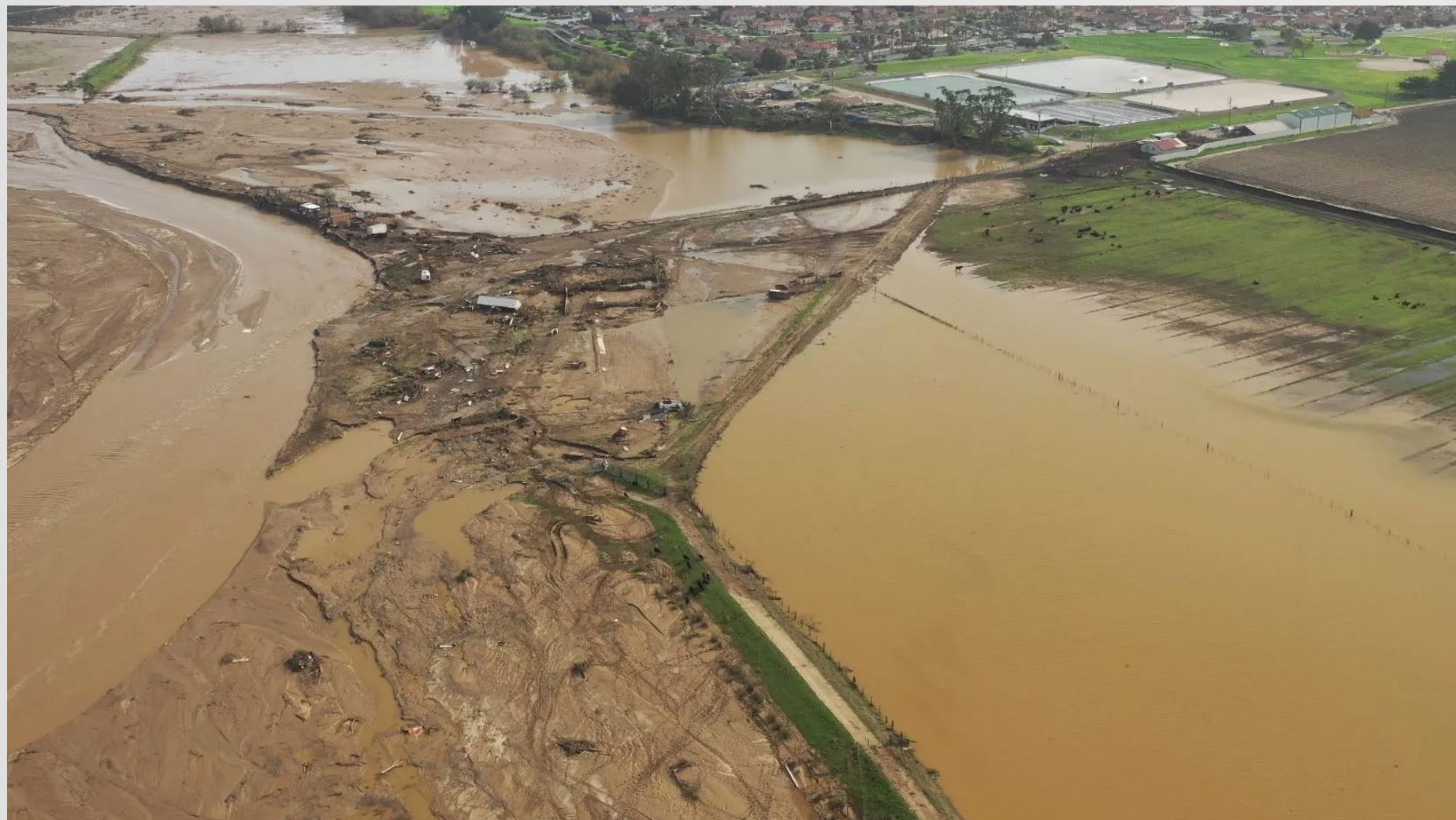
January 9, 2023, Santa Maria levee breach causing extensive flooding in the City of Guadalupe of Santa Barbara County.
