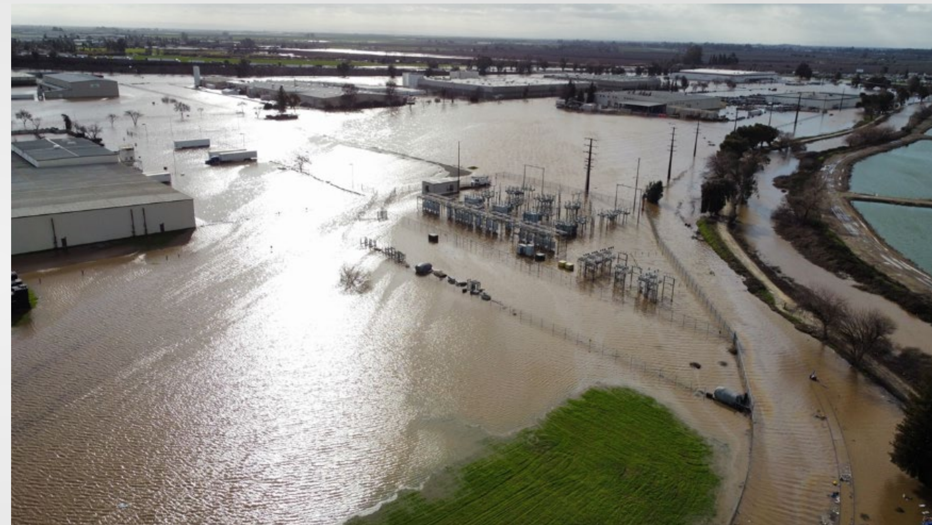
January 10, 2023, Levee break on Bear Creek in Merced, CA.
