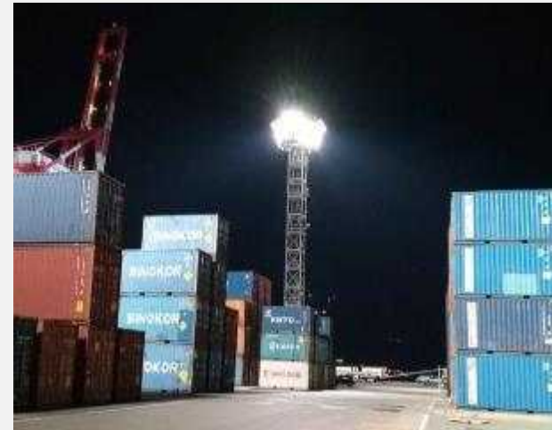
&lt; After installing LED lights &gt;
