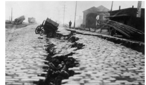
Lateral spreading cause by 1906 earthquake in San Francisco
