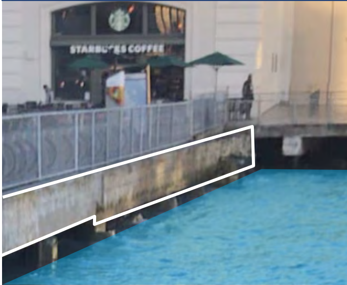
WHARF TODAY AT CURRENT WATER LEVEL
