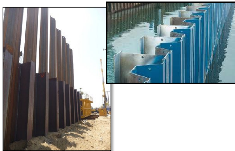
Sheet Pile Wall
