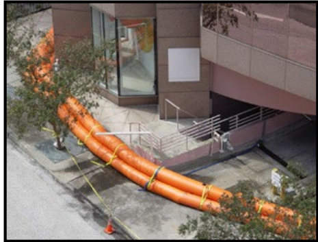
Tiger Dam: Vinyl tubes filled with water or cement slurry
