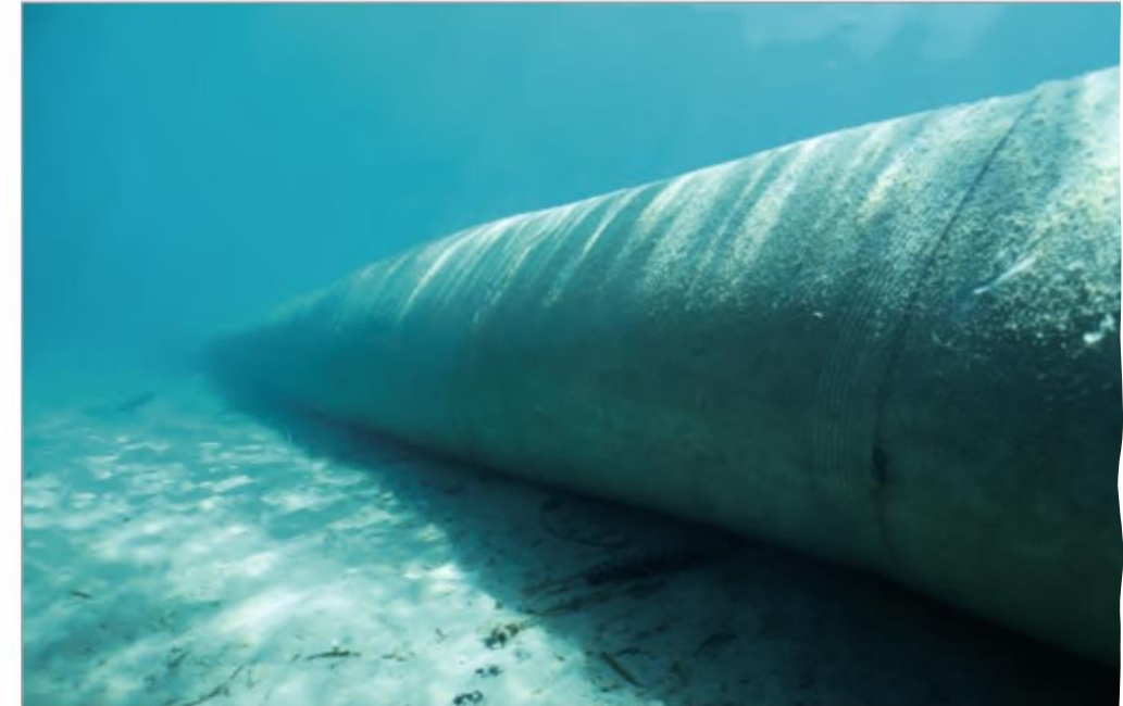
SoilTain Tube as artificial reef breakwater
