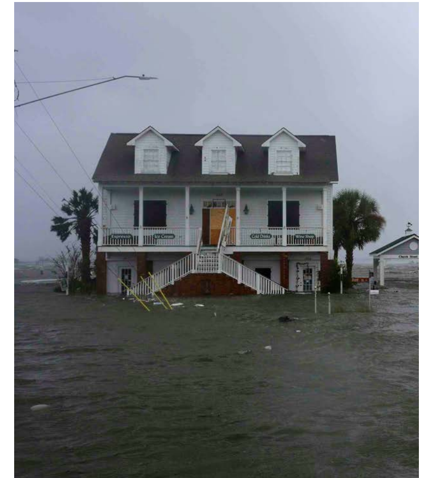
Surge flooding in Wilmington
