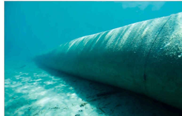
SoilTain Tube as artificial reef breakwater
