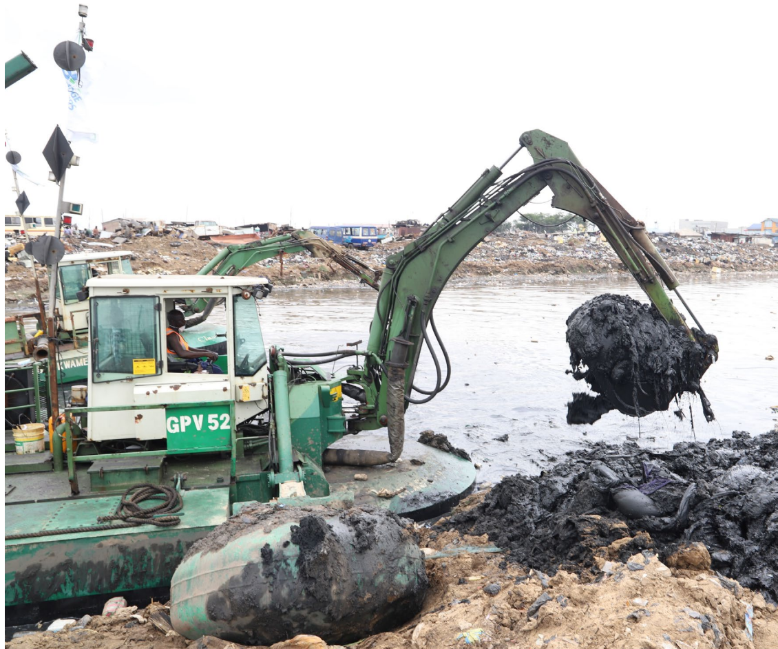
Removing the material by excavating.
