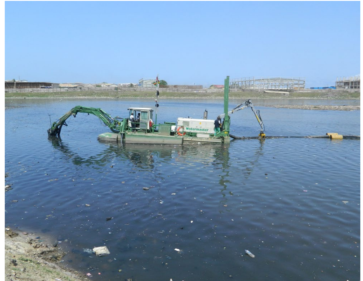
Removing the material by suction dredging.
